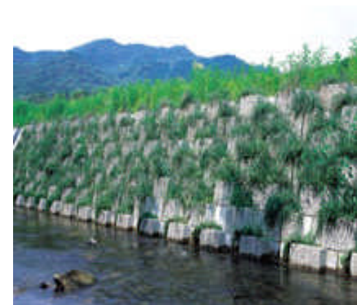
Early attempts to green the banks of flood protection works. Source: Manual for Technical Standards, 2007.
