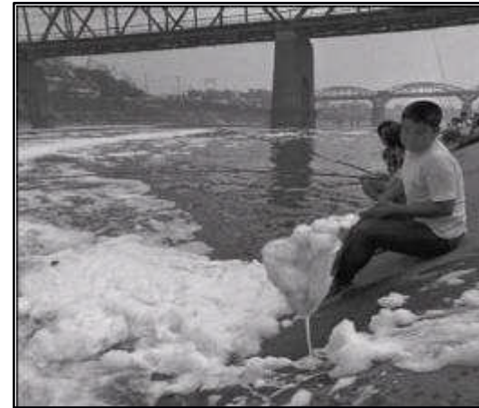
Tama River, Tokyo, 1970s Source: River Front Centre, Tokyo.
