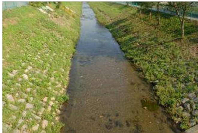
Early attempts to green the banks of flood protection works. Source: Manual for Technical Standards, 2007.
