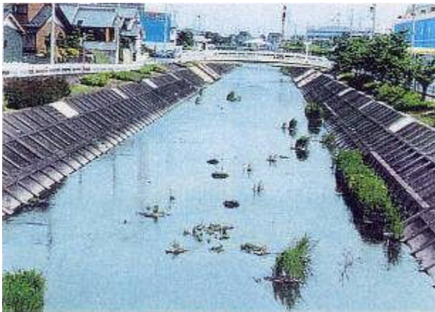
Early attempts to green the banks of flood protection works. Source: Manual for Technical Standards, 2007.
