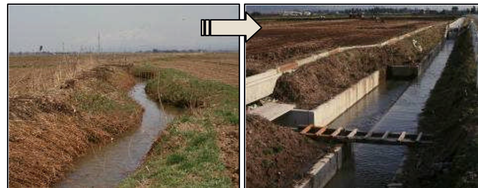
Many agricultural earth canals were built into concrete to rationalize the water usage. Source: W.W. Kelly, Japan Focus.
