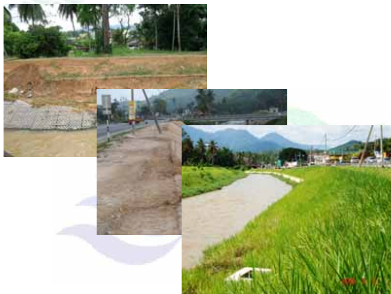
Riverbank Protection : River embankment protection w/flexible green system Sg. Bentong, Pahang
