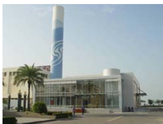
Sewerage System Museum
