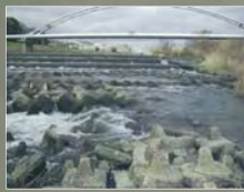
Drops on this weir is too large to go over
