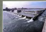
Setback type fishway Nikaryo shukugawara Dam, Tama River (出典：魚道事例集)
