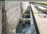
Combined fishway Ice harbor + vertical slot Arai dam, Shinano River (出典：国土交通省)
