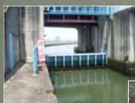
Combined fishway Ice harbor + vertical slot Arai dam, Shinano River (出典：国土交通省)
