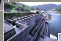
Zigzag type fishway Arase Dam, Kuma River (出典：魚道事例集)
