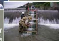
Removable fishway Chinai River ( http://www.tonuma.com/index4.html )
