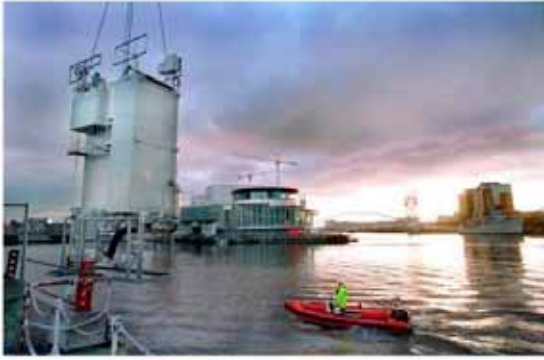
Enhancing: Through its Healthy Waterways Trust, the Campaign has promoted an innovative oxygenation project in which oxygen is pumped into a 3km stretch of the Manchester Ship Canal at Salford Quays, allowing the return of aquatic life.
