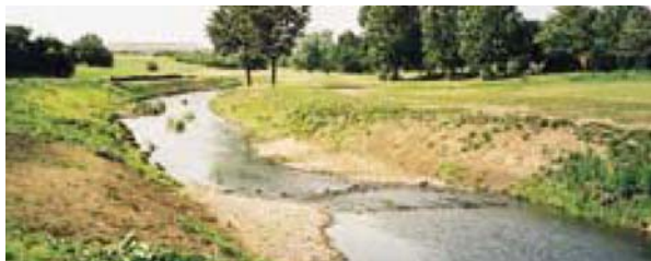
Riffles where re-meandering was not possible (The River Restoration Centre)
