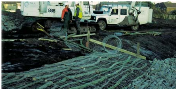
Willow mattress revetment under construction, 1995 (The River Restoration Centre)
