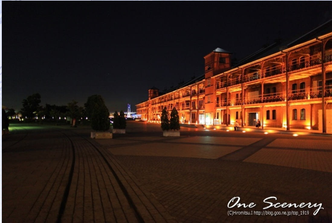
Akarenga (Red Brick) Building (Converting Warehouse to Commercial Spaces)
