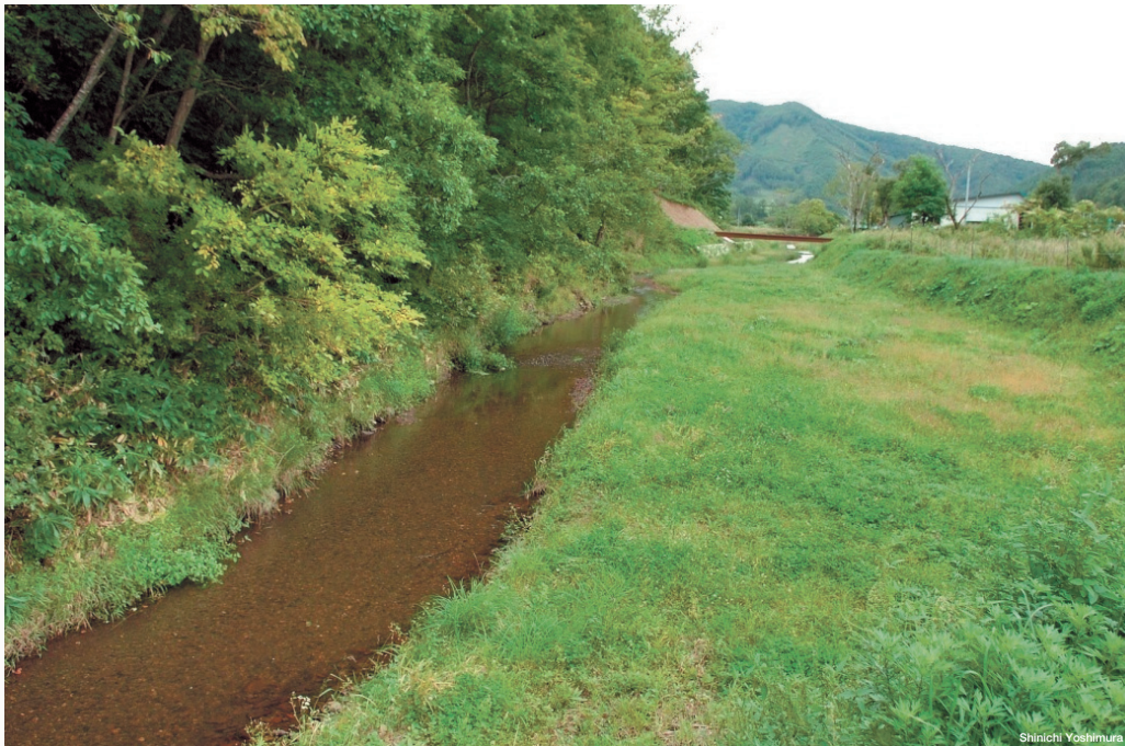
Example of one riverside widened with the mountain side conserved (Yamaya River, Japan)
