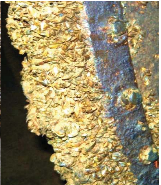
Colonization of golden mussel on concrete walls in a water transfer tunnel
