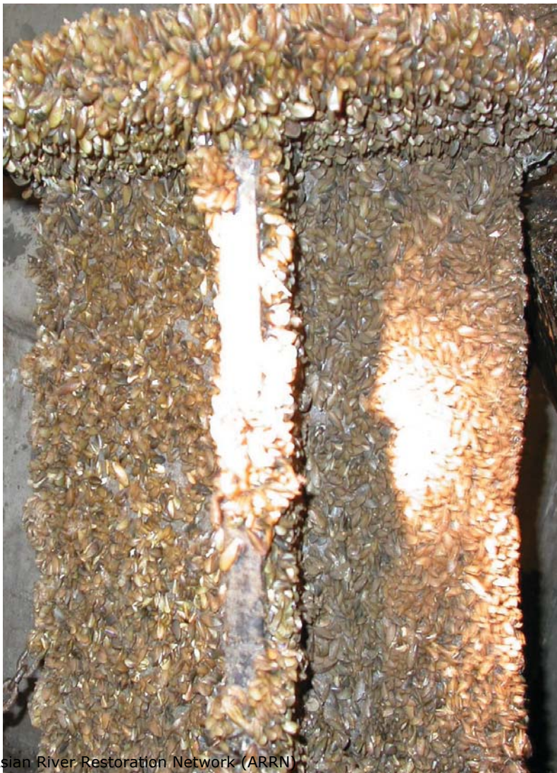
Colonization of golden mussel on concrete walls in a water transfer tunnel
