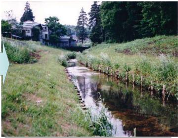
The results of extending river width, devised a revetment on shore, shallows and pools are formed.
