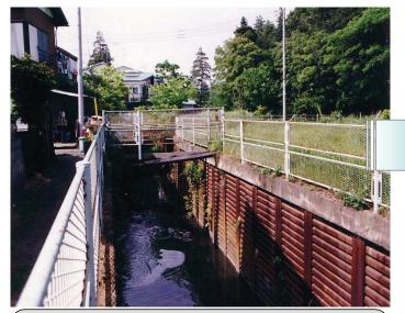
It Used to be the river with poor habitat, which river banks are covered in steel sheet pile
